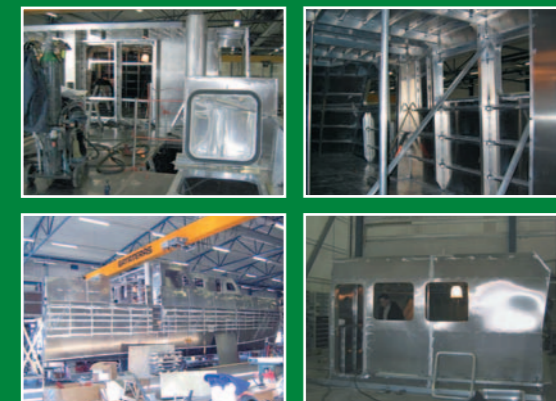
views of construction - March 2005
