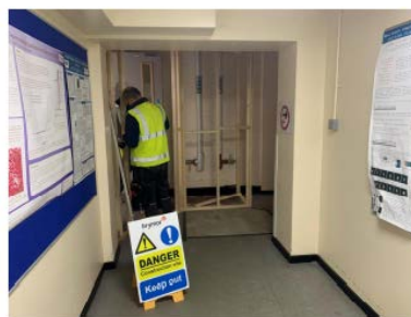
Building 27 Level 1 | Internal site hoarding being constructed within corridor 1705
