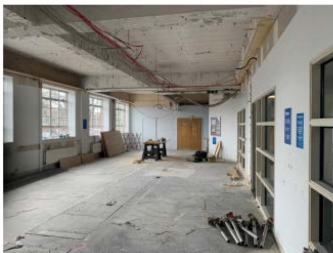
Building 27 Level 1 | Old CLS rooms stripped out
